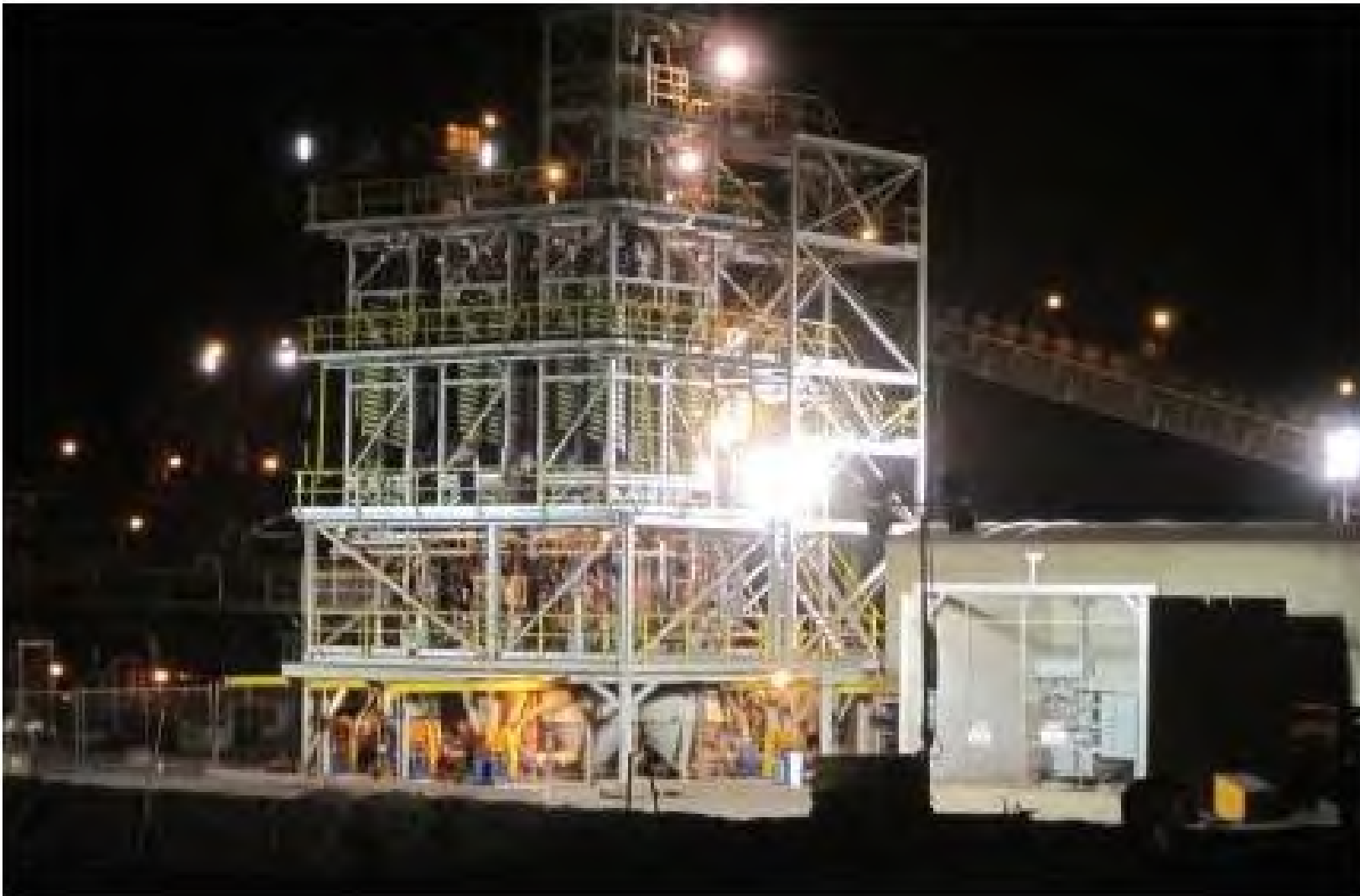
Engineering design and spiral supply to Arrium Iron Ore Project Sth Australia
