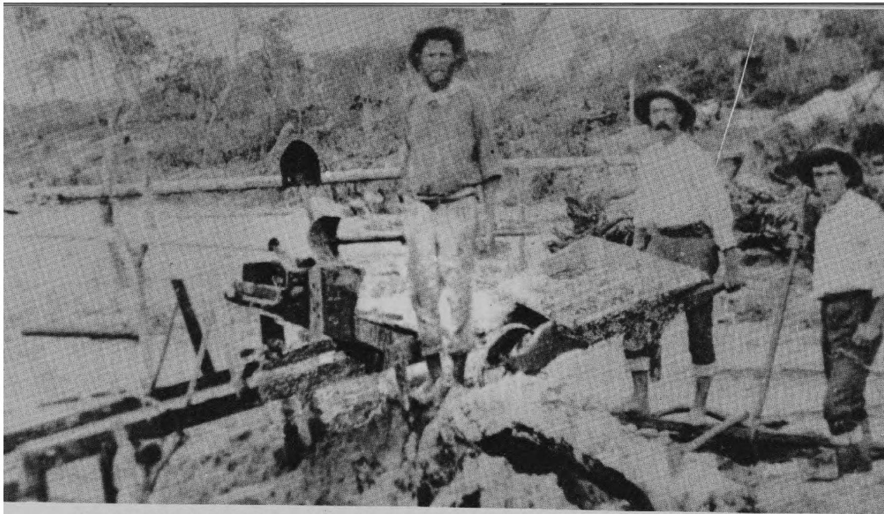
Illust. 7. Working beaches near Ballina, circa 1890. Note feeding black sand, hopper, amalgam plate, and sluice or table (carpet lined). (By courtesy Richmond River Historical Society)
