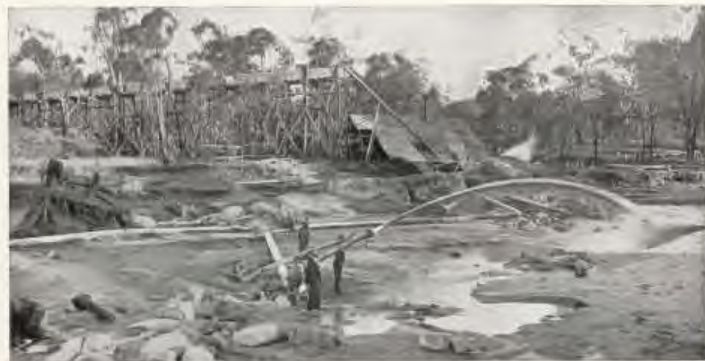
THE DREDGER AT THE ROYAL MINE, 4 miles from Stanthorpe, showing sluicing plant at work.
