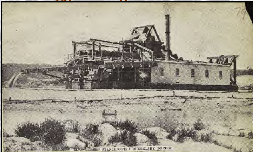
The Stanthorpe Proprietary Dredge operating on the sw portion of the Brisbane Claim in Quart Pot Creek
